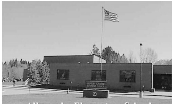
Allamuchy Township School
