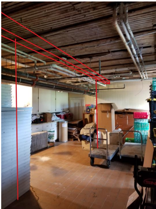
Plate 14: Below the kitchen Red lines indicate approximate location for structural reinforcing
